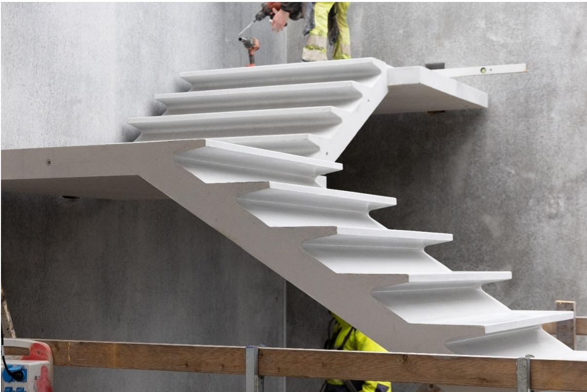
Figure 2: Ultra high strength steel reinforced concrete staircase by Hi-Con ApS.
